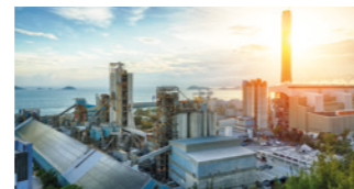
INDUSTRIAL AND STATIONARY EQUIPMENT
